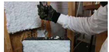
Density checks during application will ensure correct equipment calibration.
