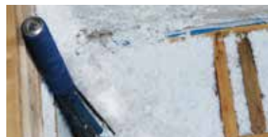
At top of cavity, reverse scrubber direction to push fiber upwards.
