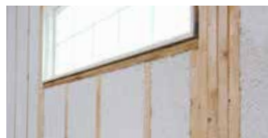
Final cavity should present a clean, well-filled appearance.
