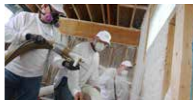
Vacuuming simultaneously with spraying will help to maintain proper moisture density.
